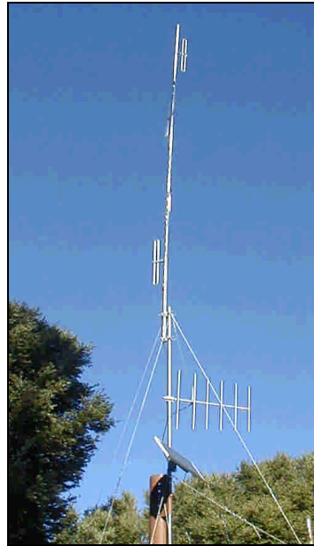
Model DB224 receive and model SAM-160 transmit antennas
